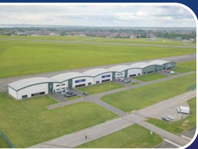
Six new hangars completed in 2018
