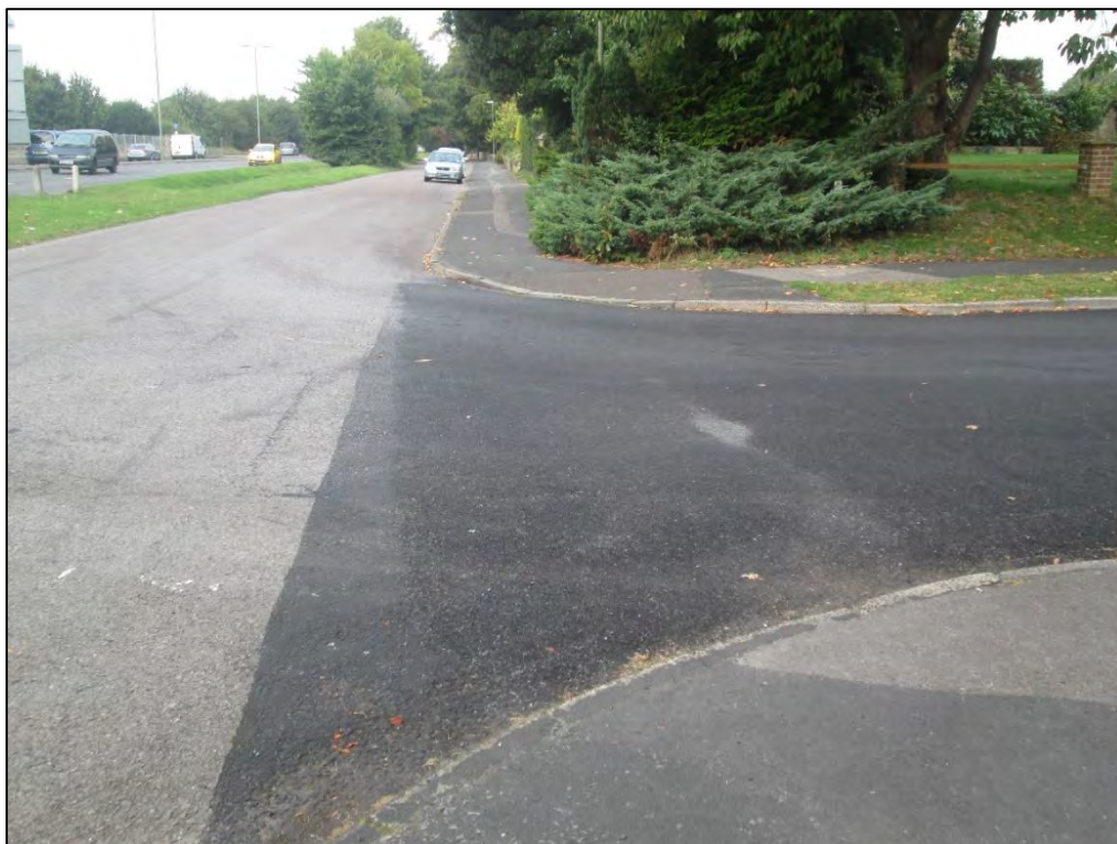
Image 2.6: No Tactile Paving at Crossing Point on Cams Hill
