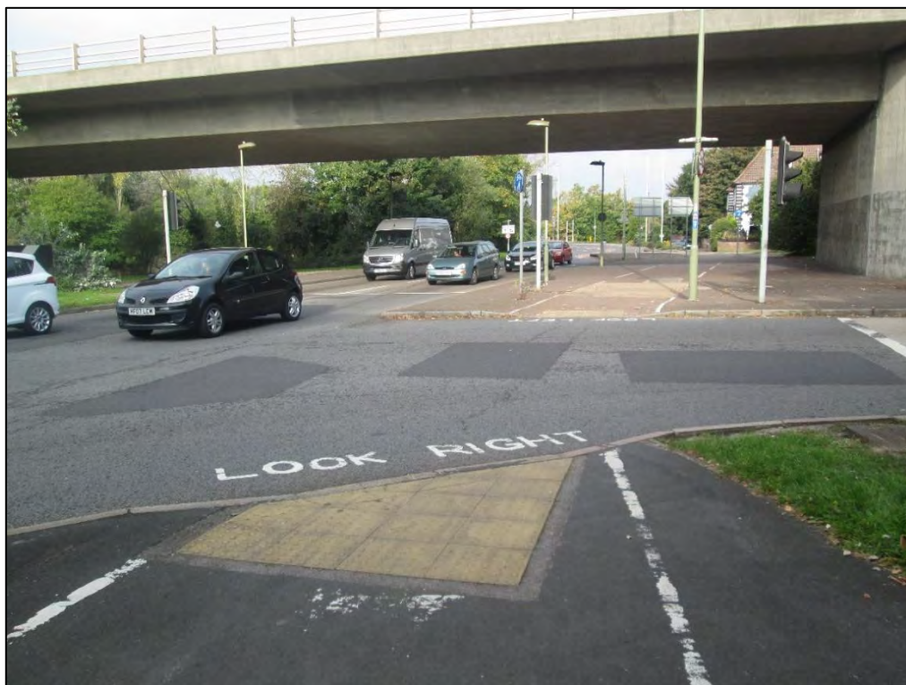
Image 2.6: No Tactile Paving at Crossing Point on Cams Hill
