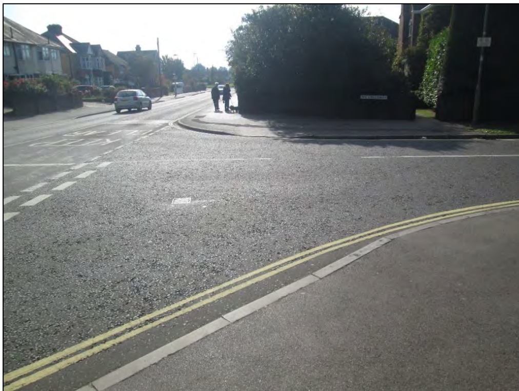
Image 4.10: Lack of Tactile Paving at The Crossway and Station Road Junction
