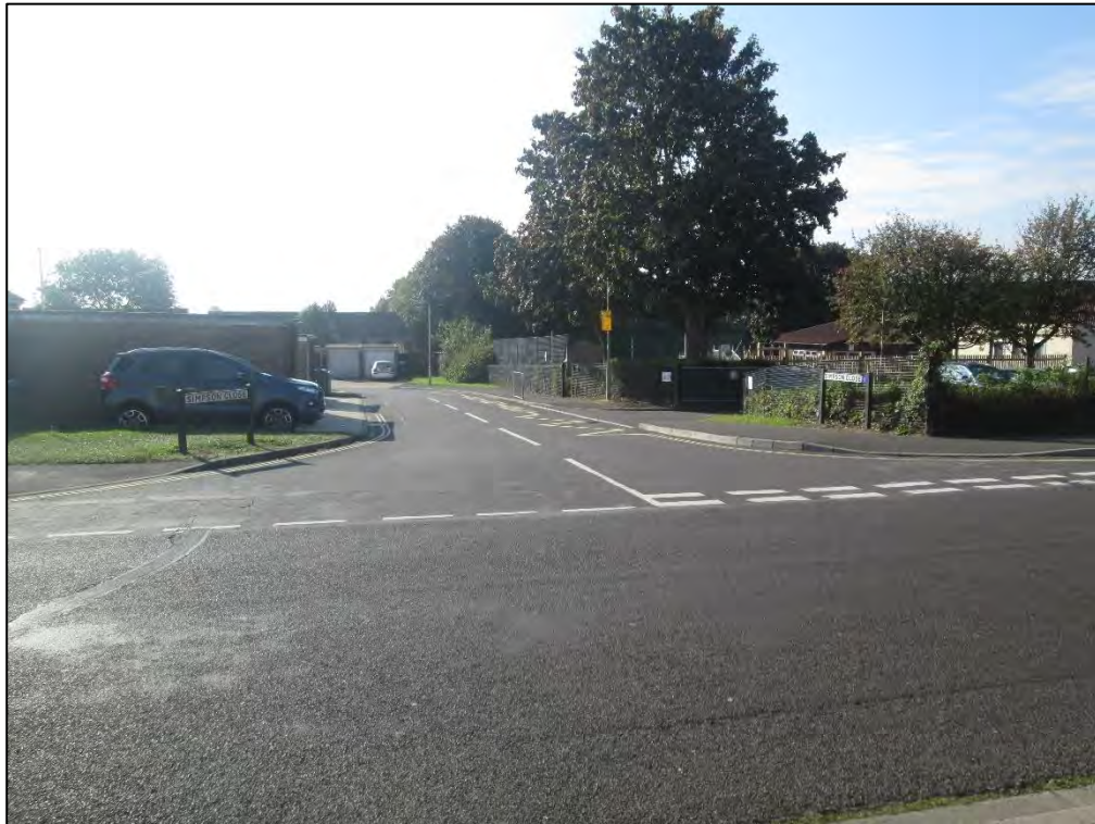
Image 4.7: Lack of Tactile Paving
