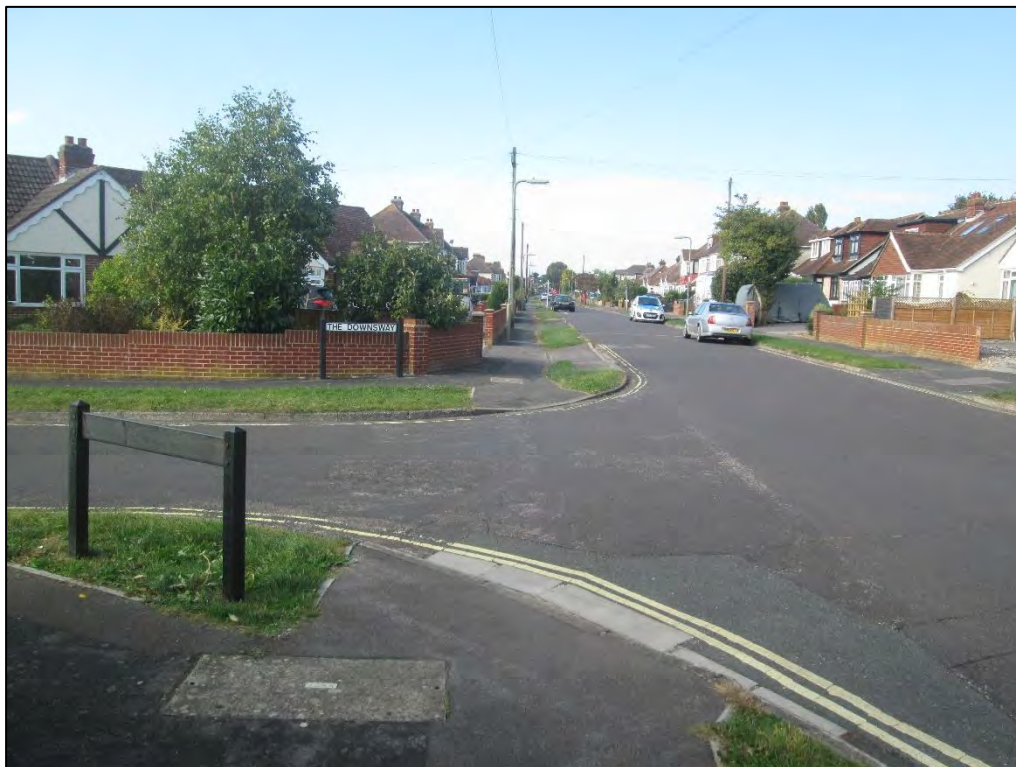
Image 4.9: Lack of Tactile Paving along The Crossway
