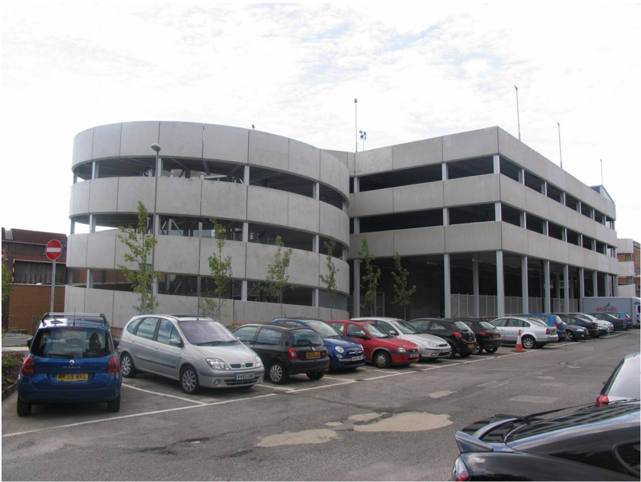
Fareham Shopping Centre Multi Storey car park
